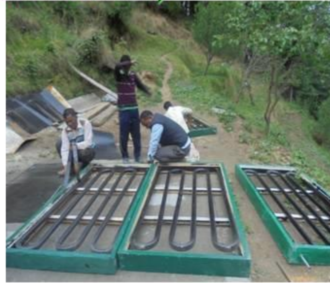
Fixing of Water Coil
